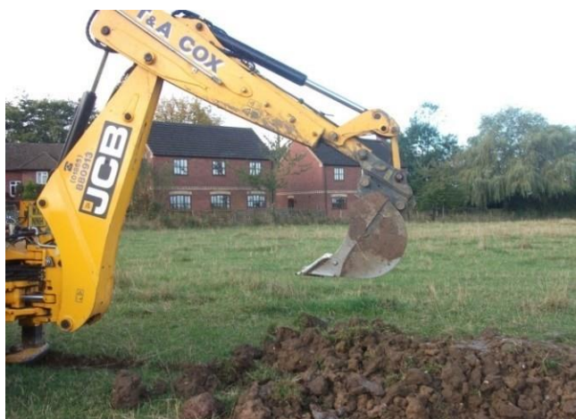
Figure 5 – Example Trial Pit
