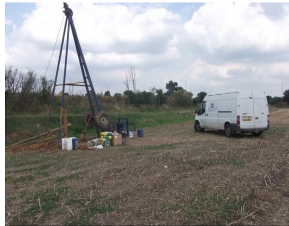
Figure 6 – Example Borehole Rig
